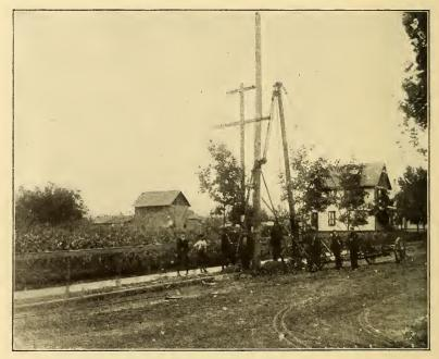
FIG. 560.-DERRICK WAGON-POLE RAISED AND BRACED.
