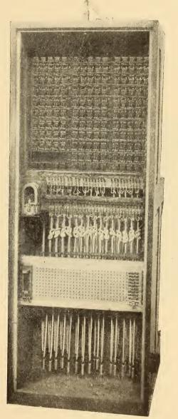
FIG. 192.-STANDARD TYPE OF SWITCH-BOARD-REAR VIEW.
