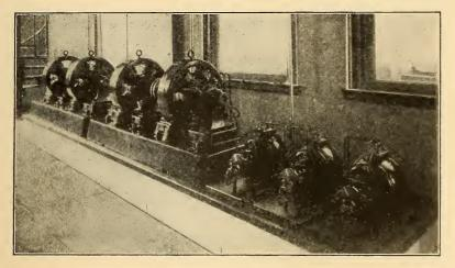
FIG. 410.-POWER TABLE-BRICK AND SLATE BASE.
