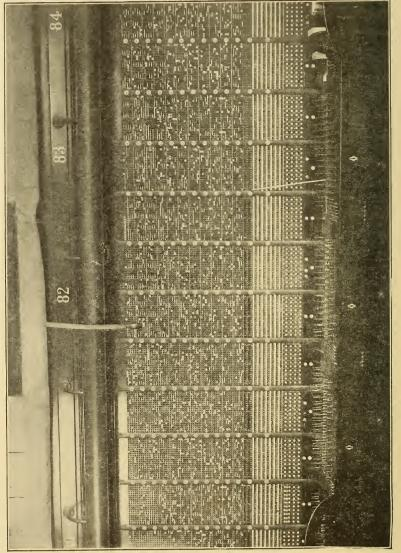
the switch-board 260 answering jacks and lamps, representing the set of subscribers' lines over which the three operators at that section receive their calls. Between the answering jacks and the mul-
