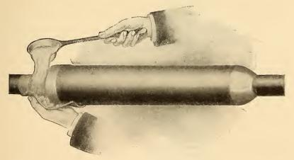
FIG. 604.—CABLE SPLICING.
