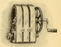
FIG. 88.-HOLTZER-CABOT THREE-BAR GENERATOR.
