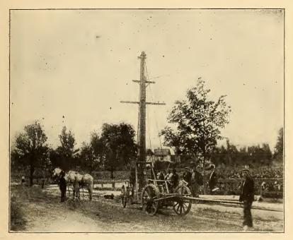
FIG. 561.-DERRICK WAGON-MOVING WAGON TO NEXT POLE,
