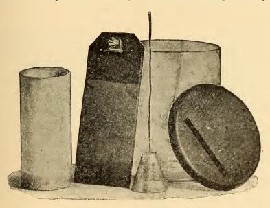
FIG. 69.-PARTS OF "STANDARD" FULLER CELL.
