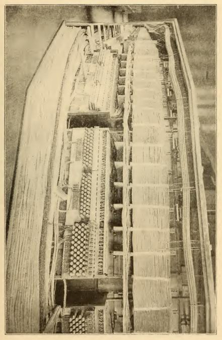
and supervisory relays, and at the bottom of the view is the mass of intermediate-to-answering cables, these cables lying in a running box on the floor, a portion of which is removed in this view for the purpose of giving a better view of the cables themselves.
