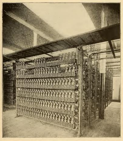
FIG. 521.—SECTION OF AUTOMATIC SWITCH-BOARD, GRAND RAPIDS EXCHANGE.
