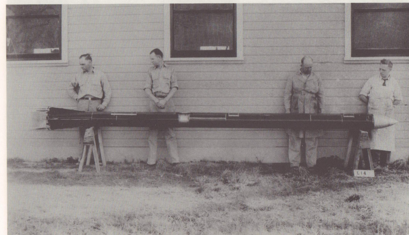
Rocket L-14's large square steering vanes were intended to insure vertical flight after burnout. Black paint was to improve visibility against dusty skies. Red quadrant is just visible along top. (courtesy of Clark University Goddard Library Archives)
