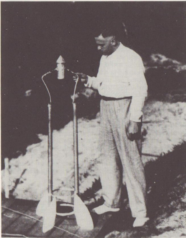
Klaus Riedel and Repulsor No. 2, a 2-Stick Repulsor with fins. (Smithsonian Institution negative no. A-4195-C)
