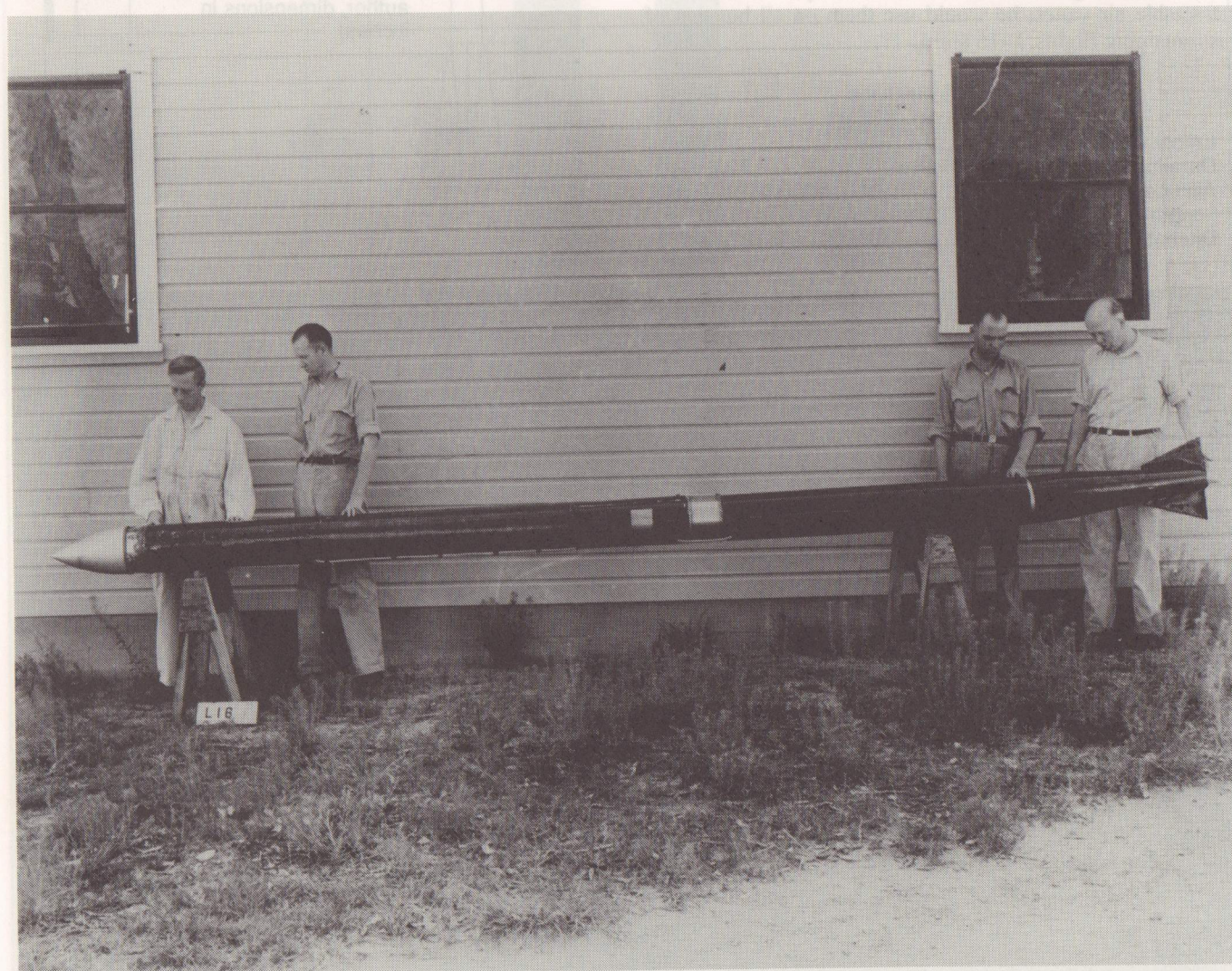
Al Kisk, Esther Goddard's brother, demonstrates the gimbaling of rocket L-16's tail section. While Robert Goddard built only one movable tail section, he felt that this would be the ultimate control mechanism for his final sounding rocket. (courtesy of Clark University Goddard Library Archives)
