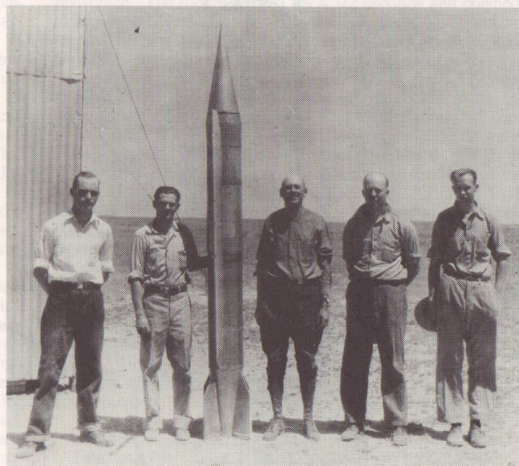
Two views of Goddard's rocket of September 29, 1931. Large fairings conceal oxygen, gasoline and pressure lines. (Left, courtesy of Clark University Goddard Library Archives; Right, NASA photo 74-H-1202)
