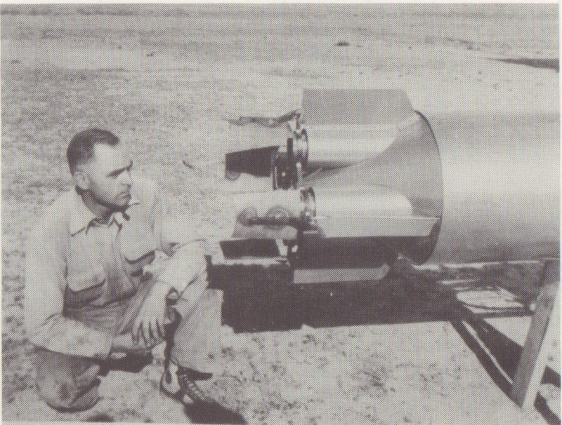
One of Goddard's crew inspects the four chambers and control vanes of Rocket L-7. (courtesy of Clark University Goddard Library Archives)
