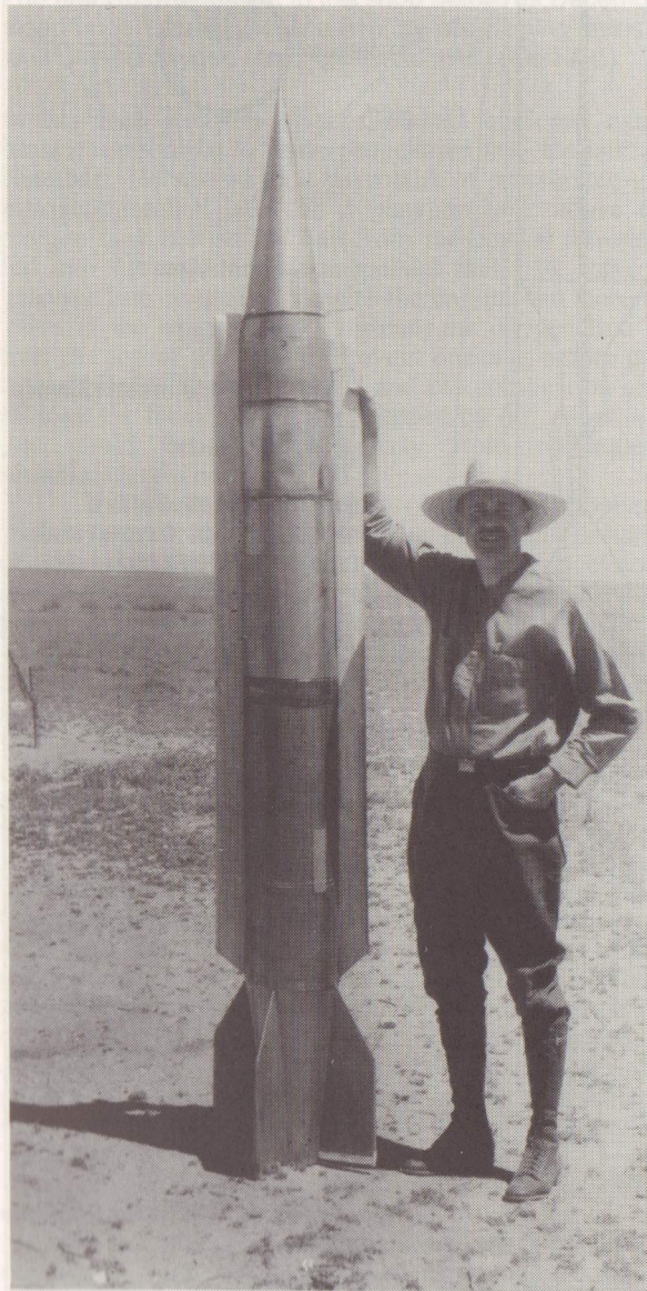
Two views of Goddard's rocket of September 29, 1931. Large fairings conceal oxygen, gasoline and pressure lines. (Left, courtesy of Clark University Goddard Library Archives; Right, NASA photo 74-H-1202)
